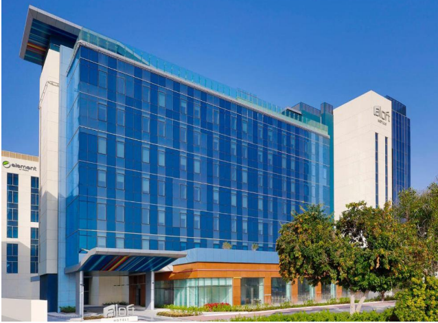
Aloft Al Mina, Dubai,UAE
